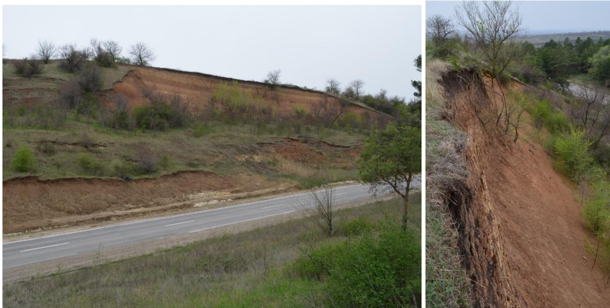
Figure 2. Deformation of the left slope of the deep excavation at PC1441+00 of the M21 road, Brest-Chisinau-Poltava Foto: Cîrlan Alexandru, April 2017.
