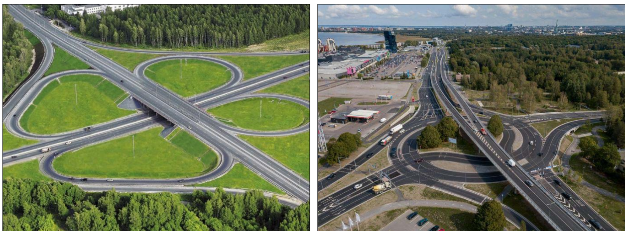
Figure 8. Auxiliary and incomplete roundabout intersections [3,16,17].
