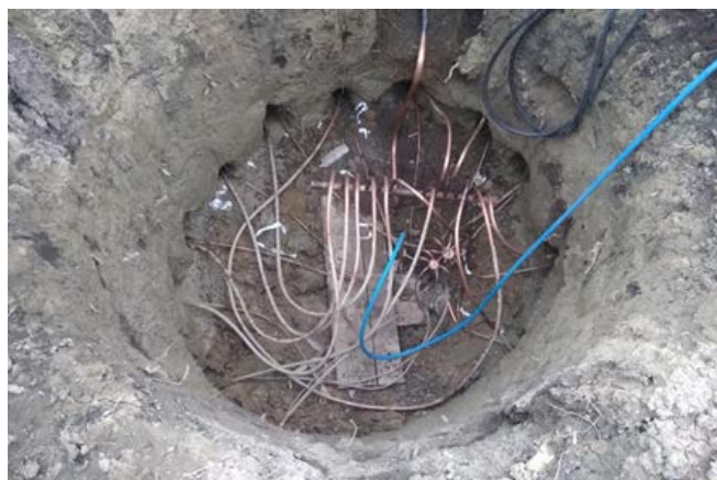
Figure 4. Geothermal circuit of the heat pump in the city of Comrat. (SRL "Climatehnic" photo)
