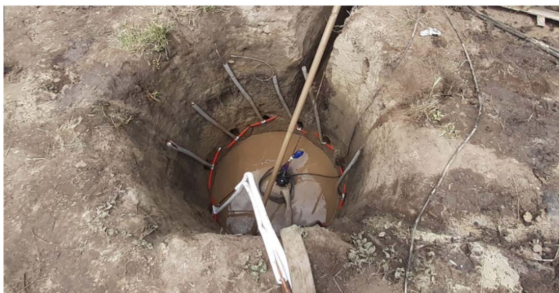
Figure 2. Geothermal circuit of the heat pump in the village of Cania. (SRL "Climatehnic" photo)
