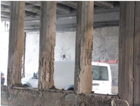
Figure 4. The Constanța Bridge pier before rehabilitation works.
