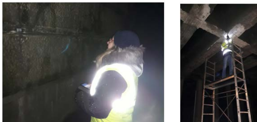
Figure 16. Data capture for structural reinforcement.
