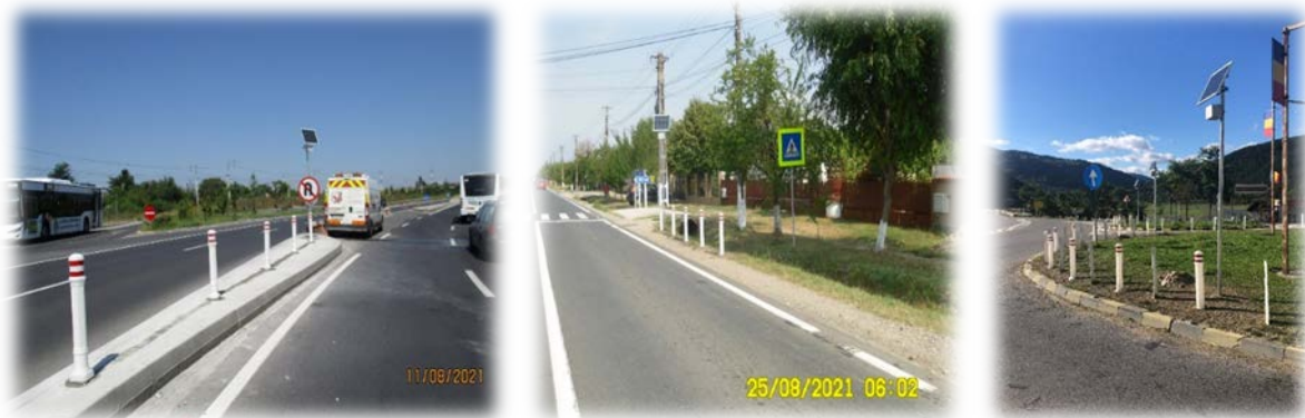
Figure 11. Lighting assemblies mounted on hazardous sectors.
