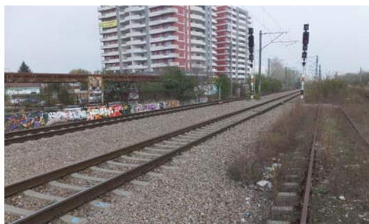
Figure 2. The railway line
